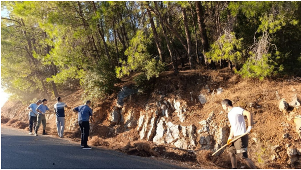
Figure 28 — Environmental clean-up on the Turunç-Amos road
